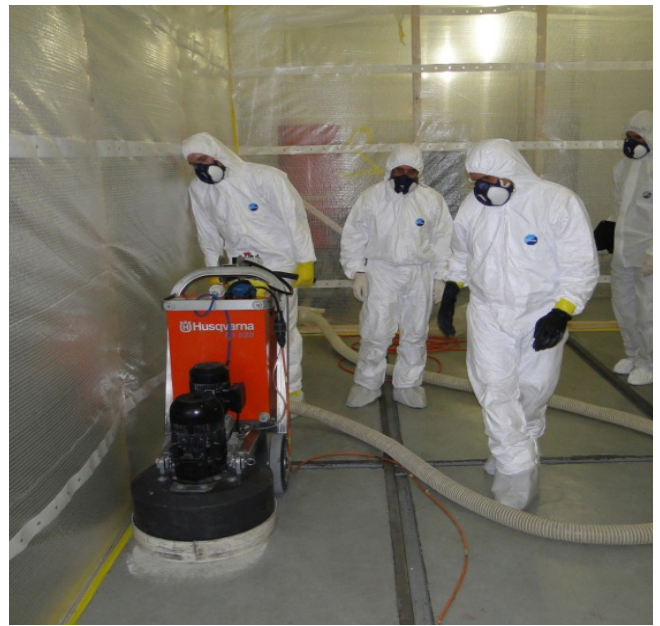
Figure 4: Removal of PCBs surface coating in industrial plant (Source ETI)
