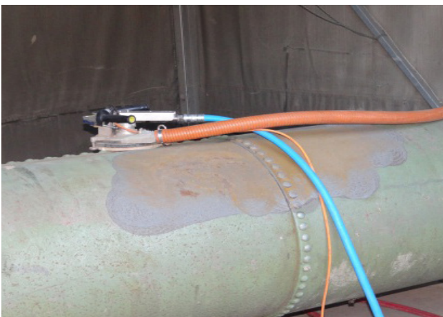
Figure 5: Decontamination of PCBs coating by high pressure water method (Source: ETI)
