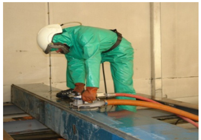
Figure 6: Decontamination of PCBs coating by high pressure water method (Source: ETI)
