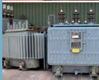
Dismantling of a PCB transformer
