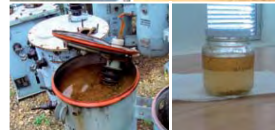
Electrical appliances with oil and water mixture
