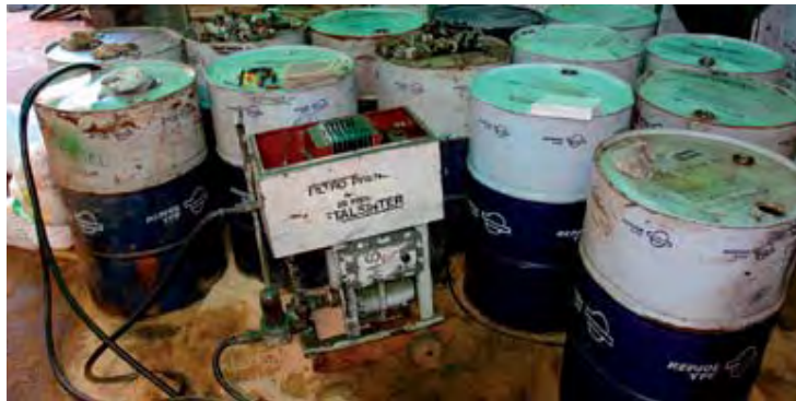
Filtering equipment of used oil, possibly contaminated
