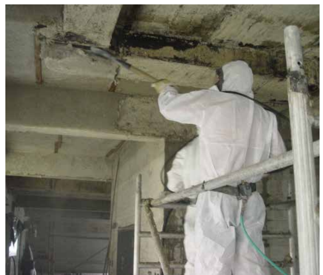
Figure 2: Removal of Sprayed Asbestos (Source: ETI [4])
