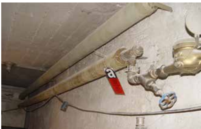
Figure 5: Labelling of asbestos containing materials (Source: ETI [4])
